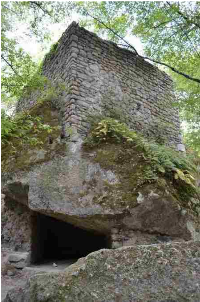
FIGURE 30 Brick tower Sacro Bosco
